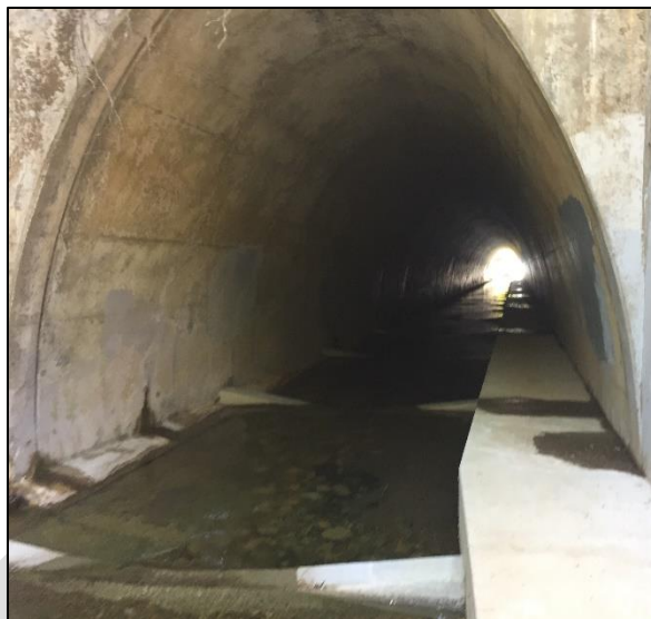
Figure 5.6-5 Drainage Under Freeway: Arroyo Hondo
